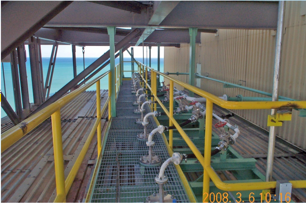
PAC Distribution Manifold
