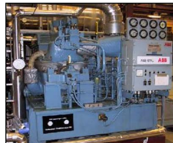
Steam Turbine Generator
