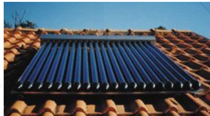
Roof Mount Tube Pumped Collector
