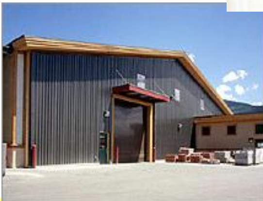
Solarwall Transpired Collector Ventilation Air Heating System
