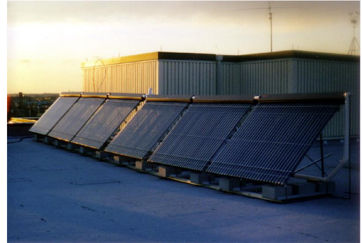
Capital Sun 360 Tube Service Hot Water Installation: Social Security Admin. Philadelphia, PA
