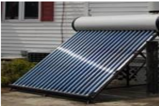
Evacuated Tube “Thermosiphon”
