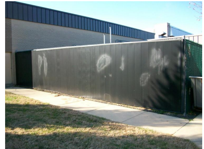
Generator Heating Collector Built on Chain Link Fence, USPS Bolger Training Center, Maryland
