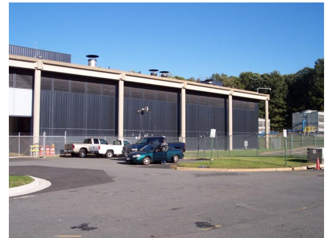
American Solar Boiler Combustion Air Heating US Geological Survey, Reston, Virginia
