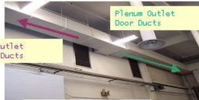
Interior Plenum Outlets
