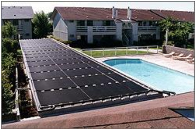
Solar Heating System with Unglazed Panels for Commercial Pool
