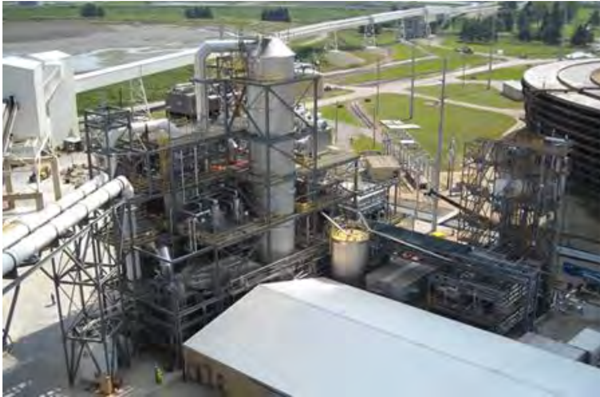
AEP Mountaineer CAP Slip Stream Plant
