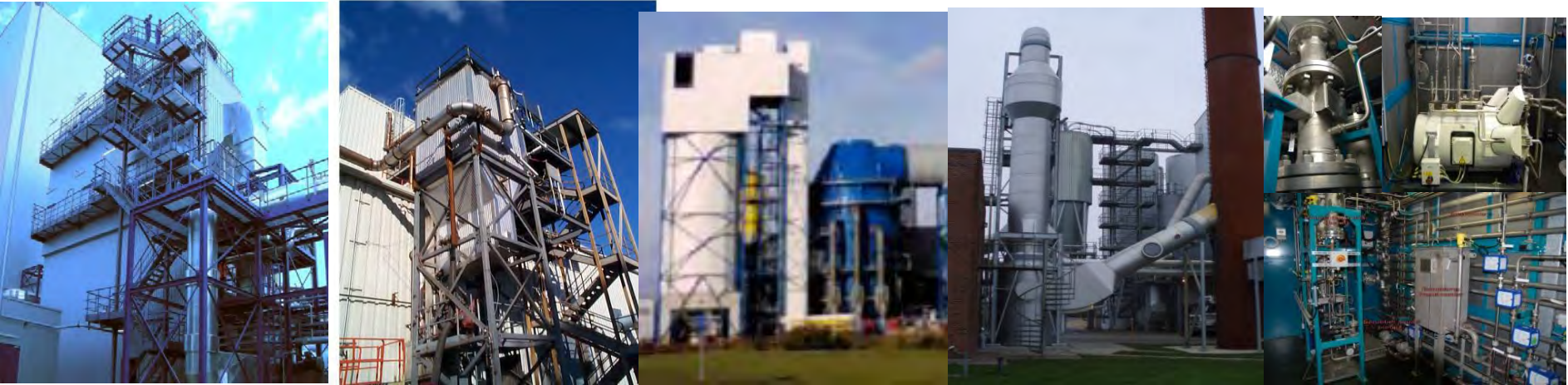
Test Equipment at Schwarze Pumpe
