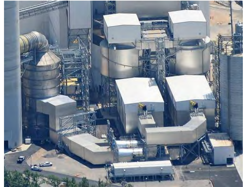
Duke Energy Cliffside Unit 6 Cliffside, NC
