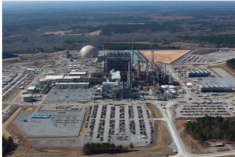
Kemper Facility – Kemper County, MS
