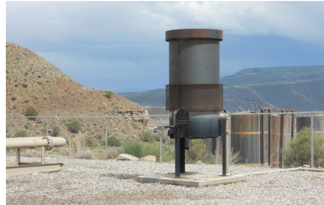
A combustion device and storage tanks. EPA photo
