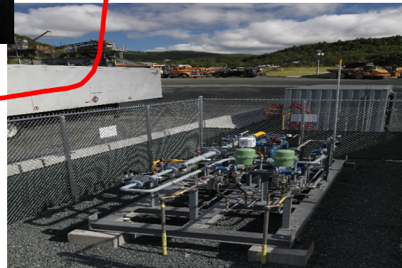
3. Customer offload facility, gas used directly from trailers
