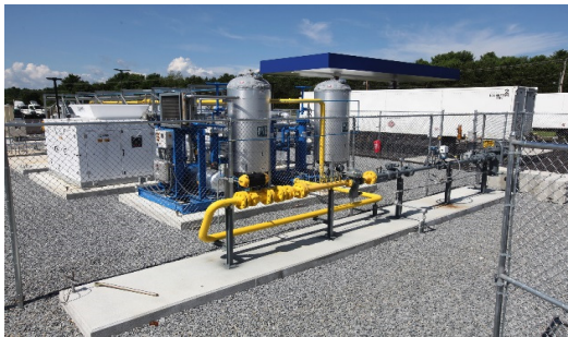
1. Compressor site on pipeline
