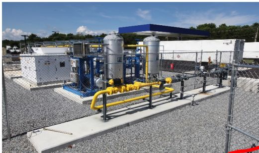
1. Compressor site on pipeline
