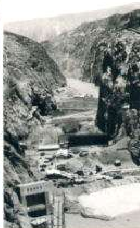
FIRST CONCRETE POURING 1933
