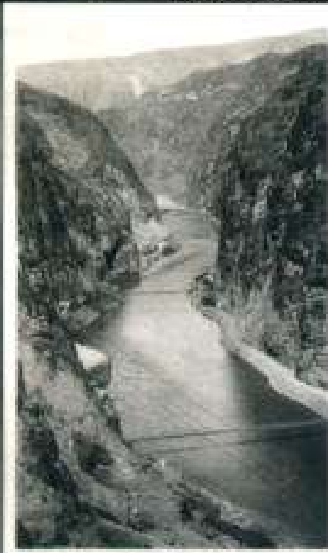
COMMENCEMENT OF CONSTRUCTION 1931
