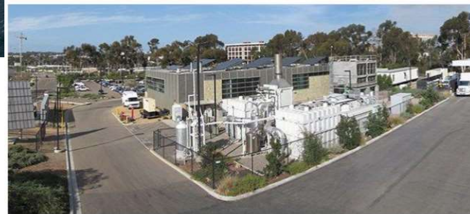
University of California, San Diego (fuel cell installed in microgrid)
