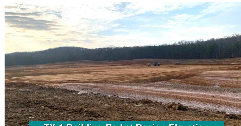
TX-1 Building Pad at Design Elevation
